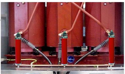
Distance line to earth part (Y) Distance to connected line (X) (parts under voltage)
